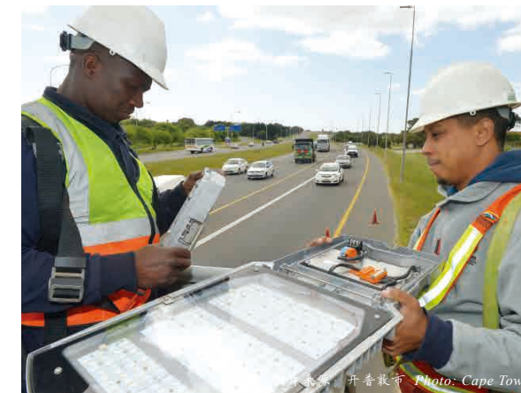
升级改造路灯 Retrofitting street lights
