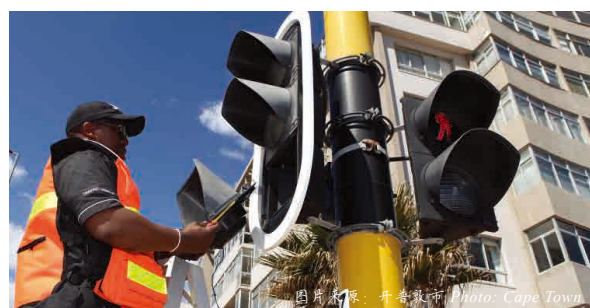
改造交通信号灯 Traffic lights being retrofitting
