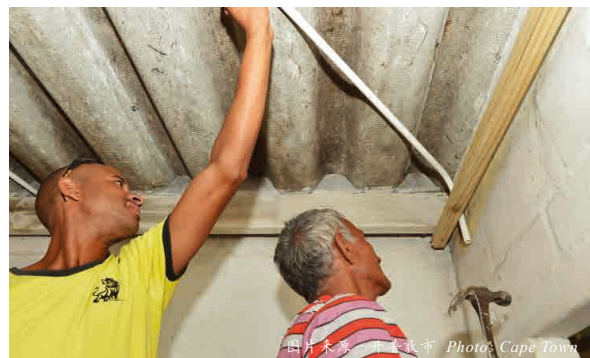
建筑屋顶翻新 Ceilings being retrofitted
