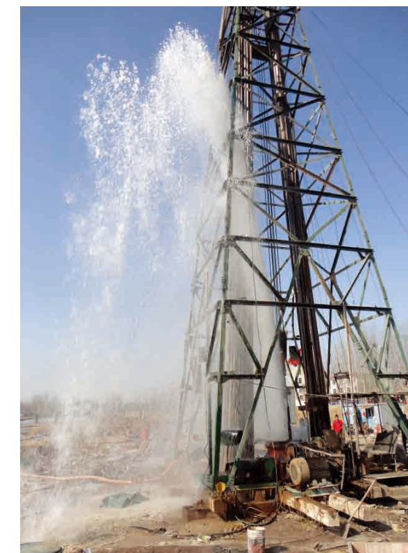
莒县店子集地热井 Ziji Geothermal Well
